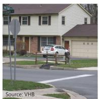
A 12-inch stop line is used to supplement the STOP sign at this residential intersection.
