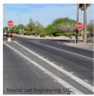
Standard reflective raised pavement markers enhance the lane lines on the approach to this intersection.
