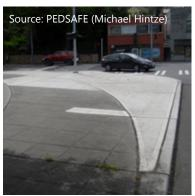
Reducing the curb radius decreases the pedestrian crossing time and distance and forces turning vehicles to slow down.
