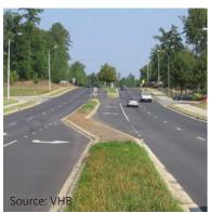
A left-turn lane removes left-turning vehicles from the through lane.
