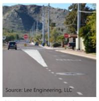
This urban right-turn lane has been installed along a stop-controlled approach.
