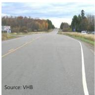
A bypass lane allows a through vehicle to pass a slowing or stopped left-turning vehicle.
