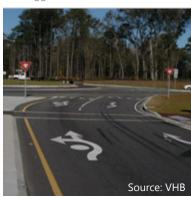
Critical guidance is provided through pavement markings along this multilane approach.
