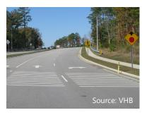
Transverse rumble strips are applied along this multilane stop-controlled approach.
