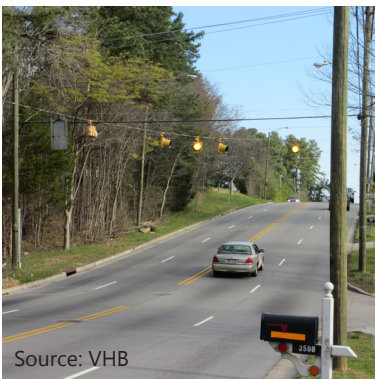
Source: VHB This Intersection Control Beacon is used at an intersection adjacent to a crest vertical curve.
