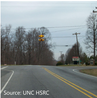
Source: UNC HSRC The Intersection Control Beacon flashes yellow from the uncontrolled approach.
