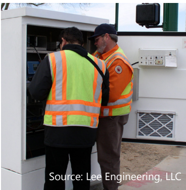
Traffic engineers adjust the timing of a traffic signal at its control cabinet.
