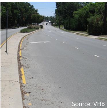
The photos above show two vantages of the same T-intersection; the top photo shows the major road left-turn lane and channelization, while the bottom photo shows the major road left-turn acceleration lane.
